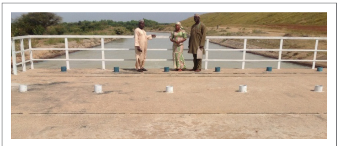
Figure 3: Upstream Tiga Irrigation Channel in Kano.
