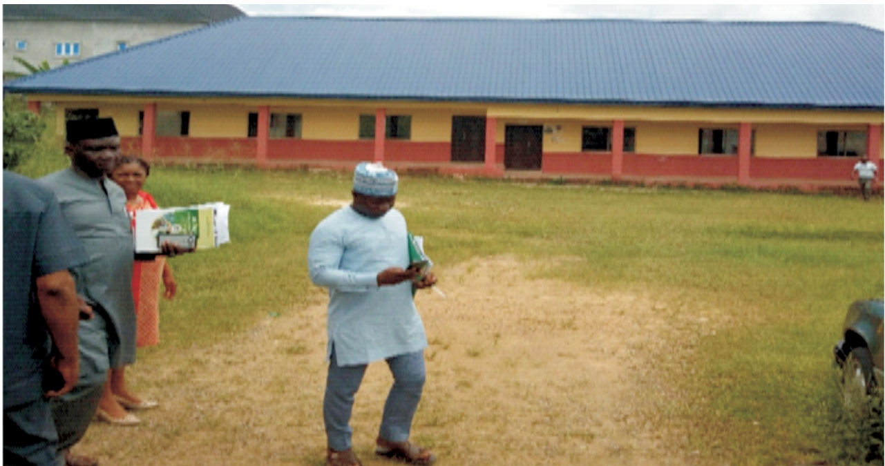
Picture 2 Completed Students' 1-Mini Student Lecture Halls, with 3 no. toilet UNICAL Teaching Hospital, Calabar (Audit)
