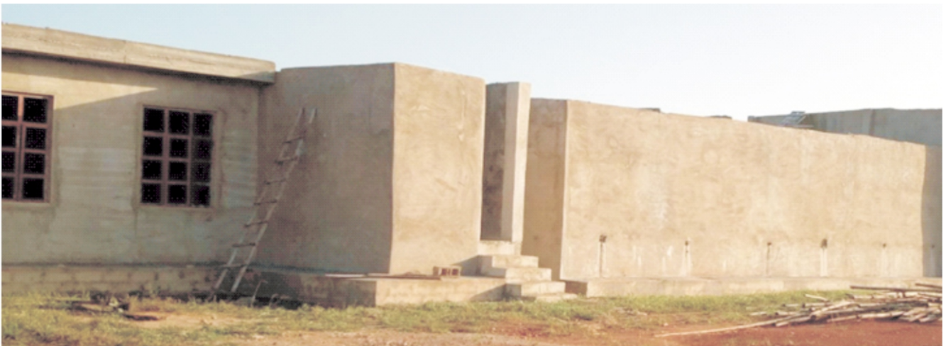
Picture 3a: Construction of Primer Cap Production Line at the Defence Industries Corporation of Nigeria (DICON).
